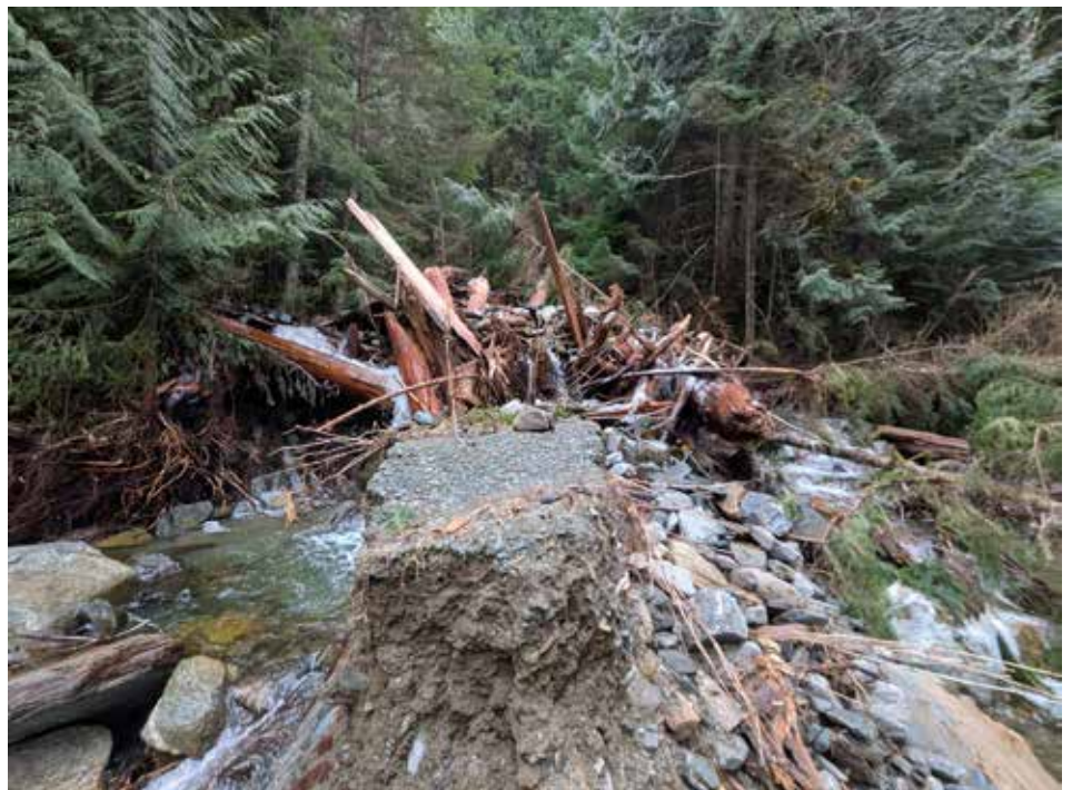
This new washout appeared on the road to the Hidden Lake trailhead, where Sibley Cr. went through an undersized culvert, after December's rain-on-snow event. More such washouts will doubtless be found as hikers start heading to trailheads this Spring.
