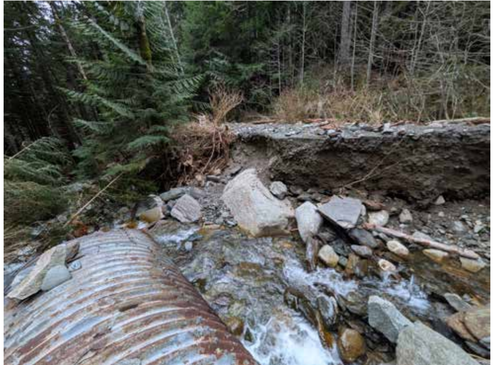
This new washout appeared on the road to the Hidden Lake trailhead, where Sibley Cr. went through an undersized culvert, after December's rain-on-snow event. More such washouts will doubtless be found as hikers start heading to trailheads this Spring.
