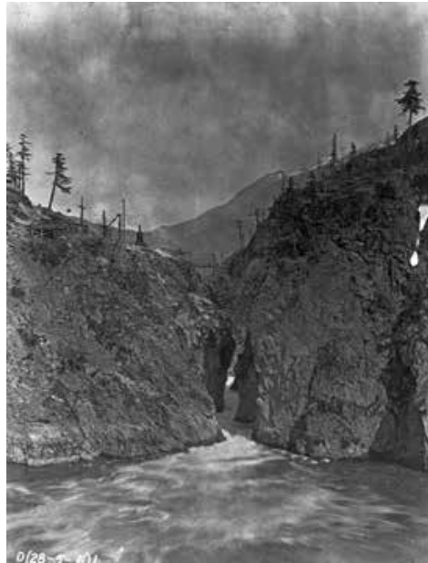
Photo 1. Skagit Gorge at the site of Diablo Dam. Note the incision of narrow (20 ft. wide) inner canyon into the broader rock valley floor above.
