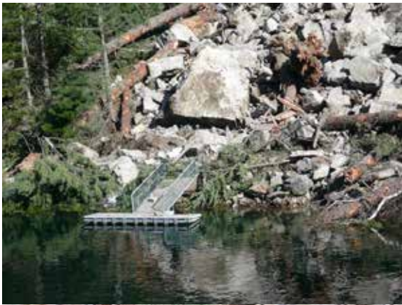
Photo 2. Debris avalanche in 2013 just below Ross Powerhouse in Skagit Gorge.
